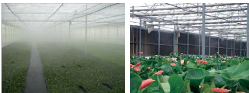
Figure 6. Evaporative cooling systems: (left) fog system, (right) fan and pad cooling system.
