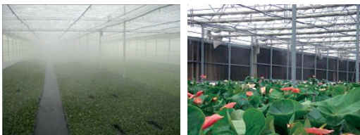
Figure 6. Evaporative cooling systems: (left) fog system, (right) fan and pad cooling system.
