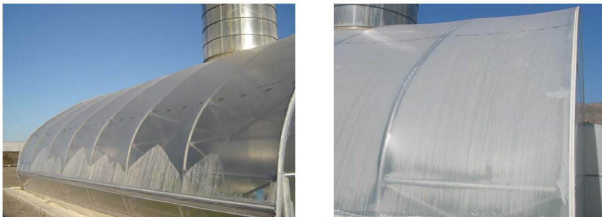
Fig. 3. Left: Image of the 5-layer plastic cover showing some spots where the anti-fog additive has disappeared. Right: Detail of the 3-layer plastic with the anti-fog property completely gone.
