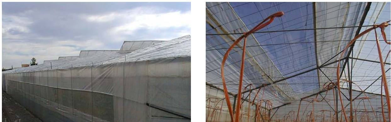
Figure 2. The two types common types of vent openings used in the Parral Greenhouse. Flap vent openings are pictured on the left and rolling vent opening on the right.
