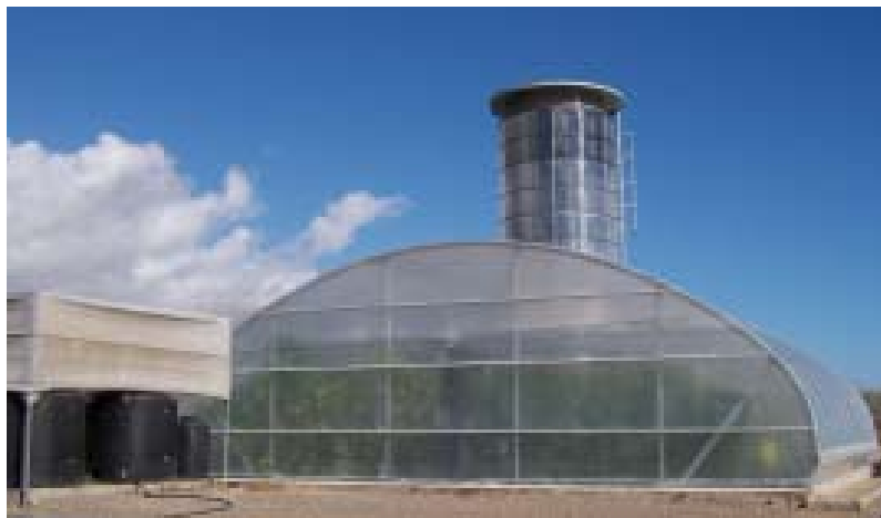
Figure 2: Watery prototype 1, built at the site of Estación Experimental de Cajamar, in Almería (Spain).
